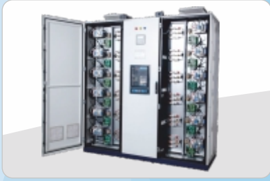
Fast Acting RTPFC Panel
