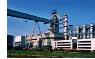
Taiyuan iron and steel (Group) Co., Ltd.
