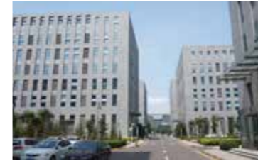
Beijing Kehua Zhongsheng Network Cloud Computing Engineering Company Project
