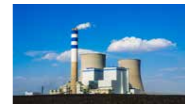
Xinjiang Hami Power Plant
