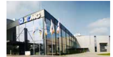
Construction Upgrading and Expansion Project of XCMG
